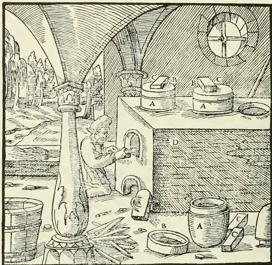
A—POTS. B—LIDS. C—STONES. D—FURNACE.
